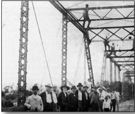
The first bridge spanning the Alafia River, connecting the early settlements of Peru and Riverview, built circa 1900. The impressive ironwork was formerly used on the Lafayette Street Bridge in Tampa with the wooden floor of the bridge "raised" to allow riverboats and steamers passage. Dr. G. H. Symmes, Peru's first medical doctor, is pictured 8th from left.
